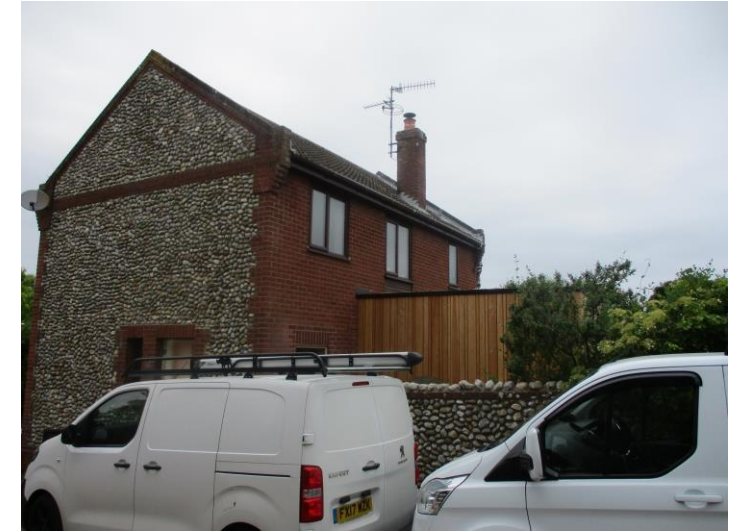
EXISTING SOUTH ELEVATION (SIDE) – FOLLOWING ADDITION OF EXTENSION
