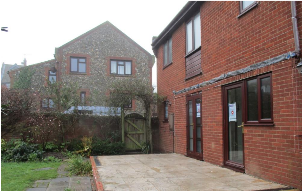
NORTH ELEVATION (SIDE) – FOLLOWING DEMOLITION OF CONSERVATORY
