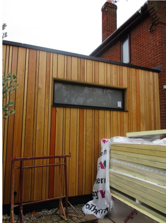
EXISTING NORTH ELEVATION (SIDE) – FOLLOWING ERECTION OF EXTENSION
