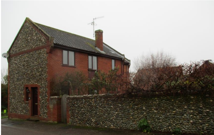
SOUTH ELEVATION (SIDE) – FOLLOWING DEMOLITION OF CONSERVATORY
