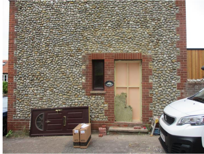
EXISTING SOUTH ELEVATION (SIDE) – FOLLOWING REMOVAL OF DOOR
