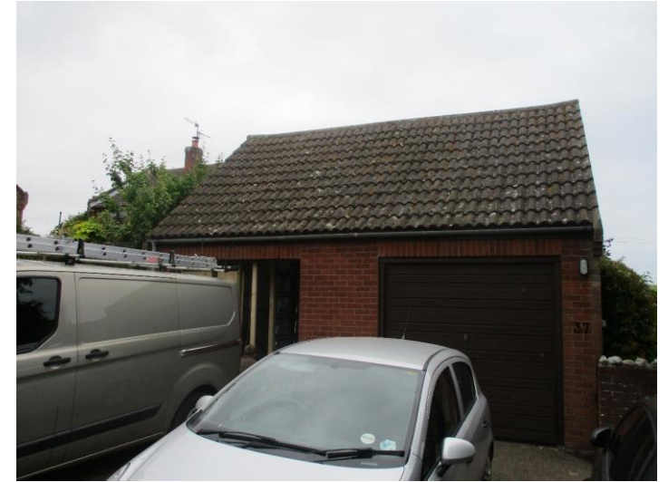
EXISTING EAST ELEVATION (REAR) – FOLLOWING REMOVAL OF GARAGE DOORS
